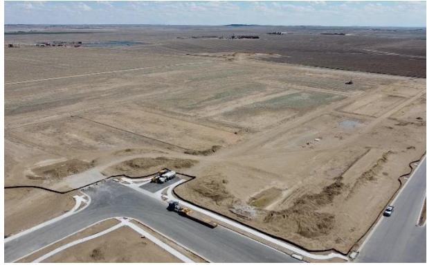
Filing 5 (View: Southeast)
