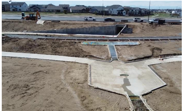
Pond C Outlet Structure (View: West)
