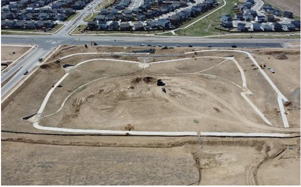
Pond C (View: West)
