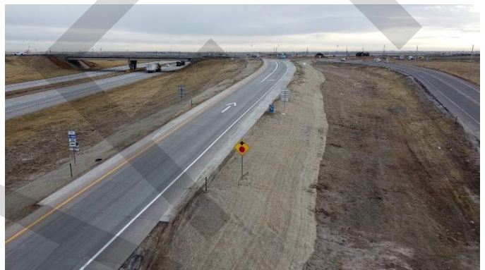
Offsite Improvements I-70 Offramp (View: East)
