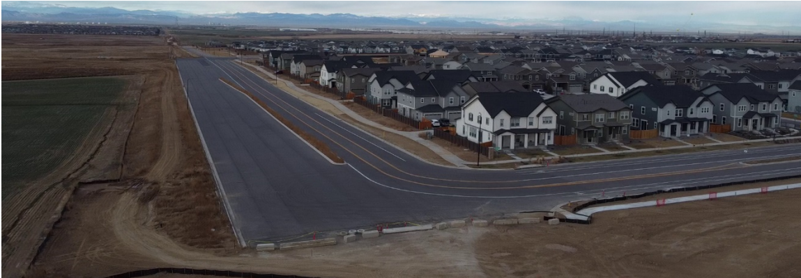
Filing 4 (View: Northwest)
