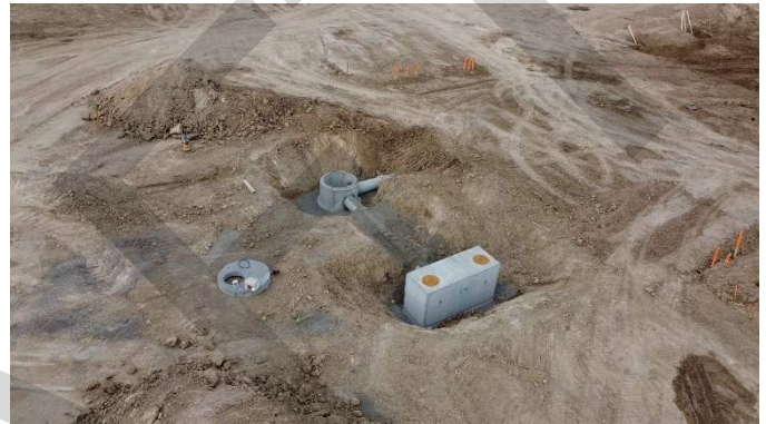
Filing 5 Installed Inlet and Manhole (View: West)
