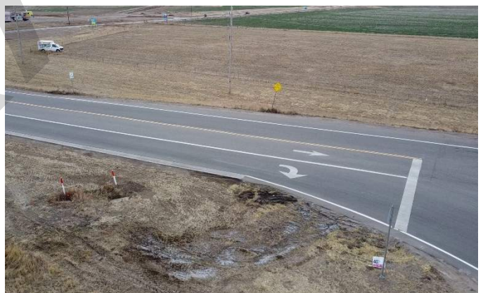
Offsite Improvements I-70 Offramp (View: South)
