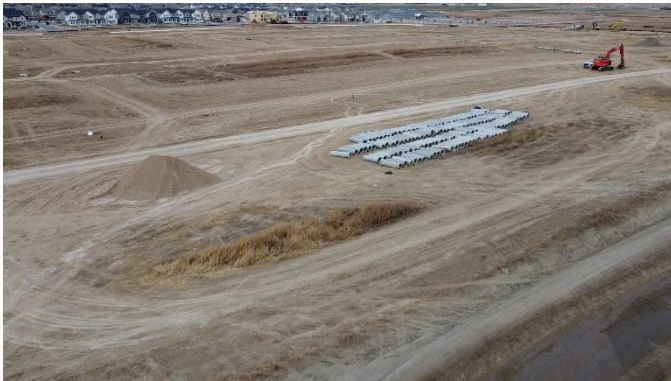
Filing 5 Tract I (Materials Stored on Site) (View: Northeast)
