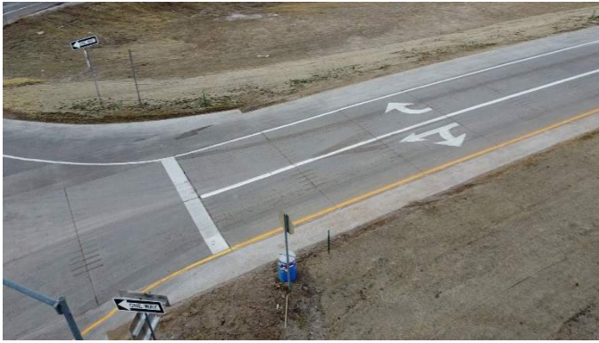
Offsite Improvements I-70 Offramp (View: South)
