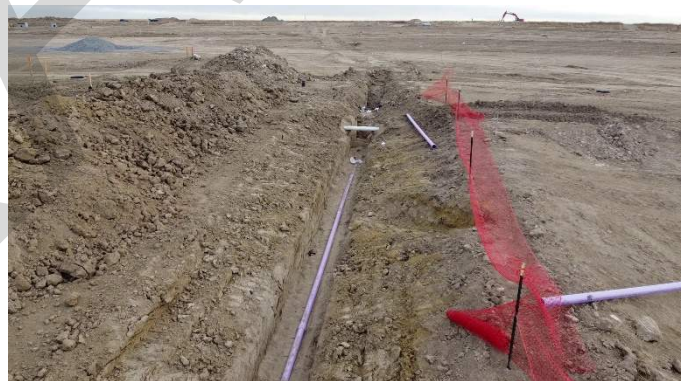
Filing 5 Installed Irrigation Pipe (View: East)
