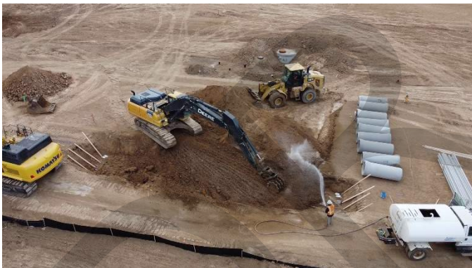
Filing 5 Installation of Storm Sewer (View: South)
