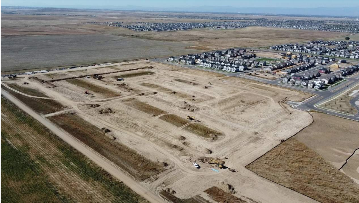
Filing 5 (View: Southwest)
