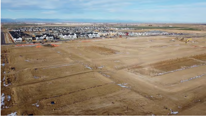
Filing 5: Overview (View: Northwest)
