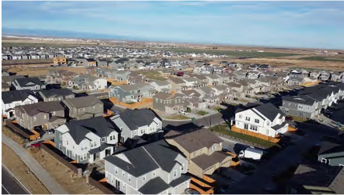
Filing 4: Overview (View: Northwest)
