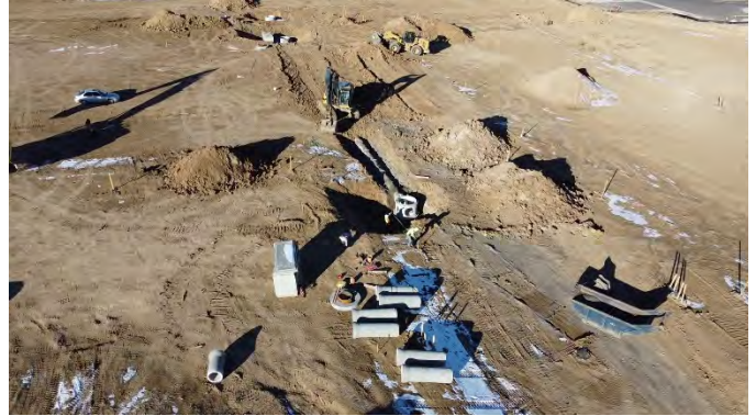
Filing 5: Storm Sewer Installation (View: West)
