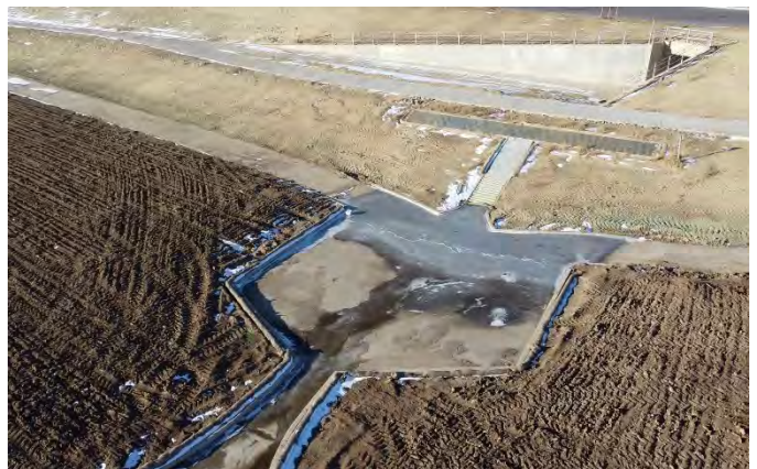
Filing 4: Tract C (View: Southwest)
