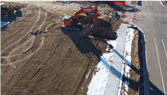
Filing 5: Excavation for Water Service (View: South)
