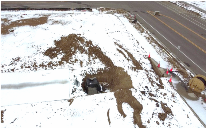
Filing 5: Tract K Drainage Improvement (View: West)
