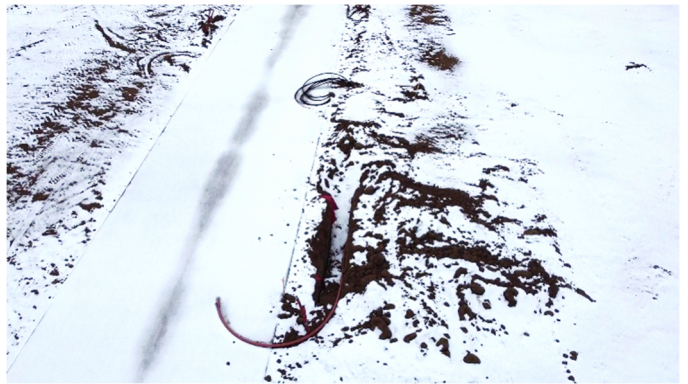
Filing 5: Conduits by Tract F (View: South)
