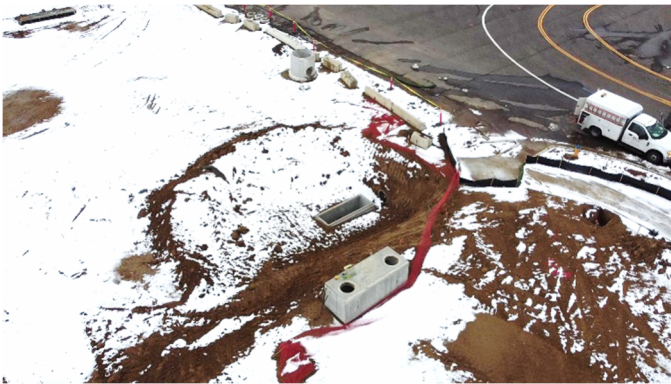
Filing 5: Storm Sewer Materials (View: Southwest)
