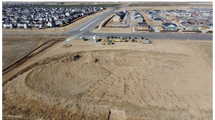
Filing 6: Tract G (View: North)
