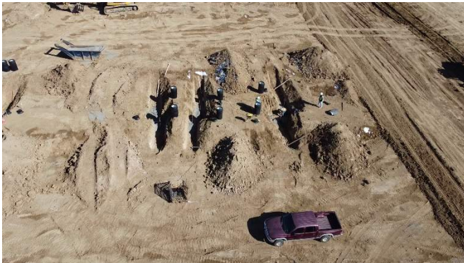
Filing 5: Water Service Installation (View: East)
