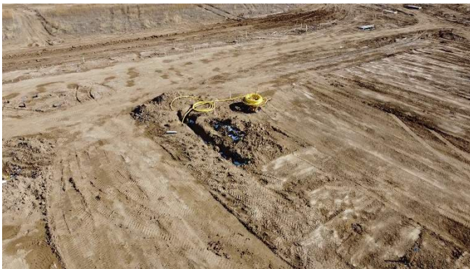
Filing 5: Sleeving installation (View: Southeast)
