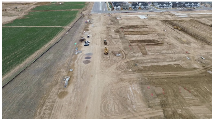
Filing 5: Future N Del Ray St and Stored Materials (View: South)
