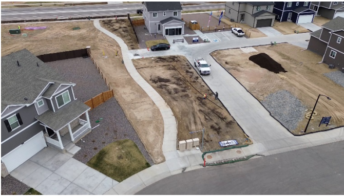
Filing 4: Tract F Steel Edger Installation (View: North)
