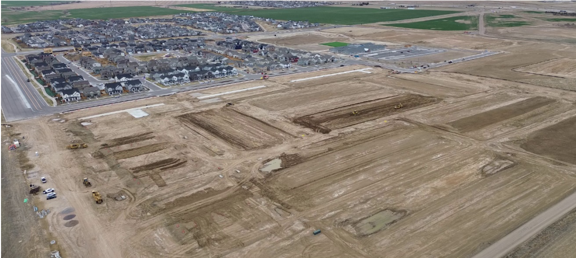
Project Overview from Filing 5 (View: Northwest)
