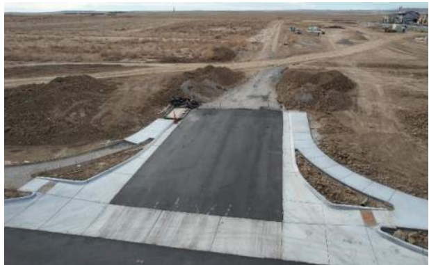
Carrie St (View: South)
