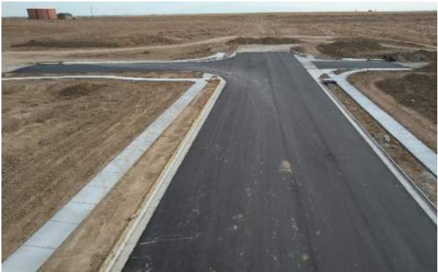
E 8th Place and Carrie St (View: East)
