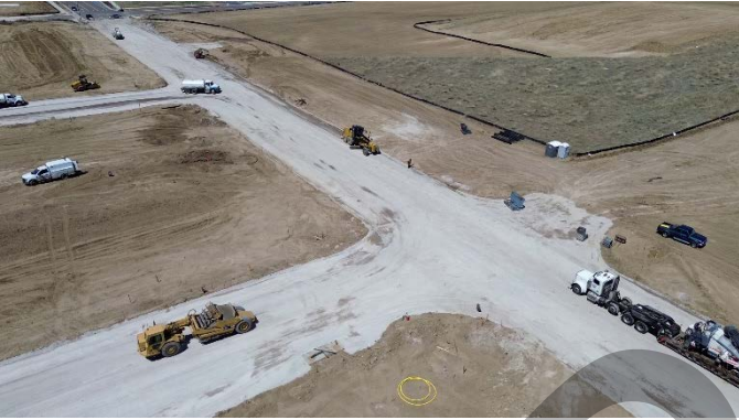
Filing 5 8th PI (View: Northeast)
