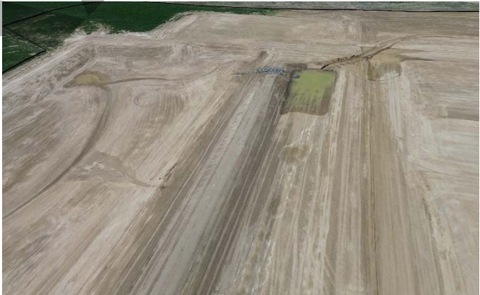
Filing 6 Tract H (Detention Pond) (View: West)
