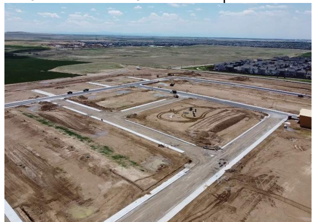
Tract B and Tract C Improvements facing Southwest
