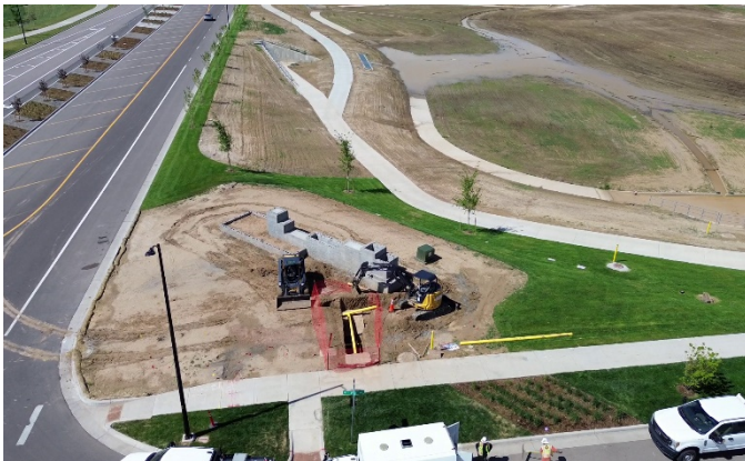
Filing 4: Monument Installation (View: North)
