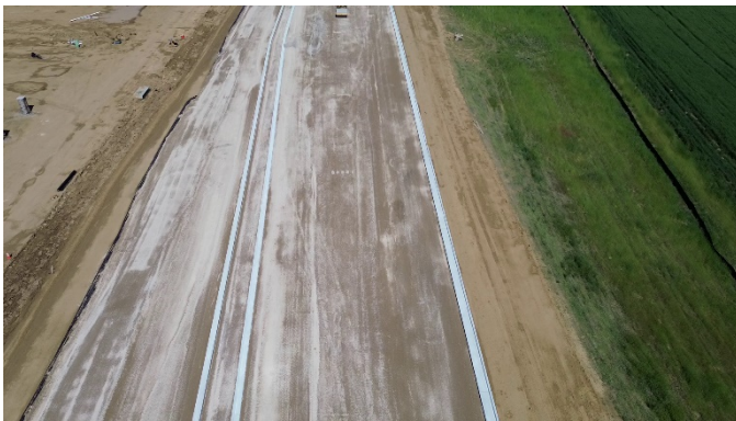
Filing 5: E 6th Ave Median and Curb (View: East)
