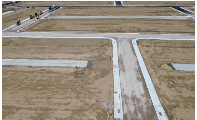
Filing 5: E 7th Pl (View: East)
