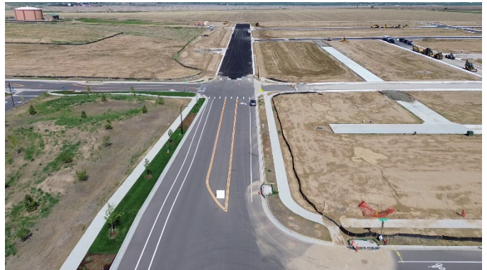
Filing 4 & 5: E 8th Pl (View: East)
