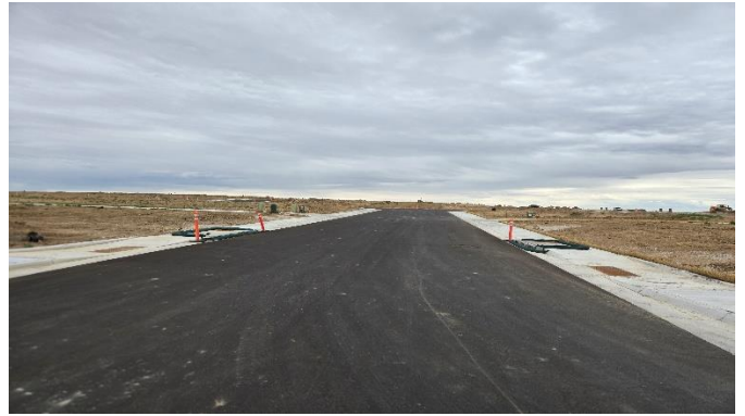
Filing 5: E 8th Ln (View: East)
