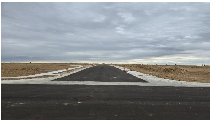
Filing 5: E 7 th Ave (View: East)
