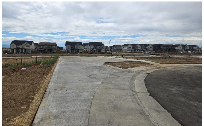
Filing 5: Tract M, E 6 th Pl (View: West)
