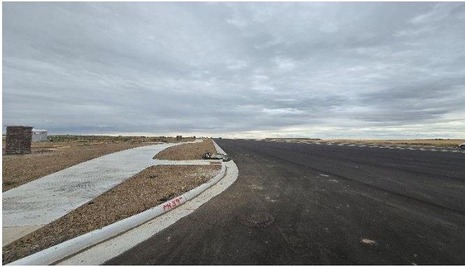
Filing 5: E 6 th Ave (View: East)
