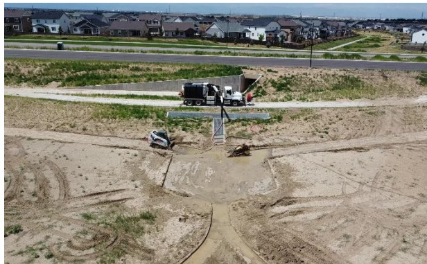
Pond C (View: West)
