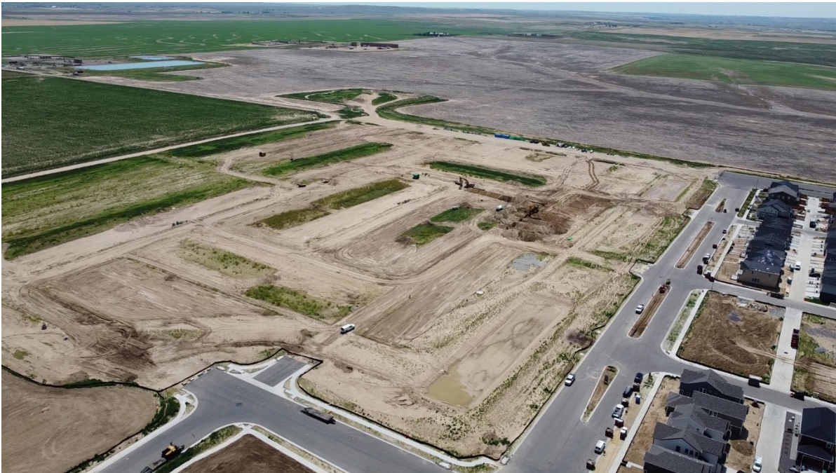
Filing 5 (View: Southeast)
