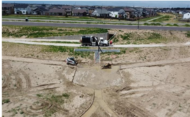
Pond C (View: West)
