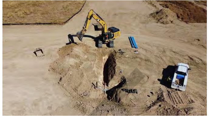
Filing 5 Wet Utility Improvements
