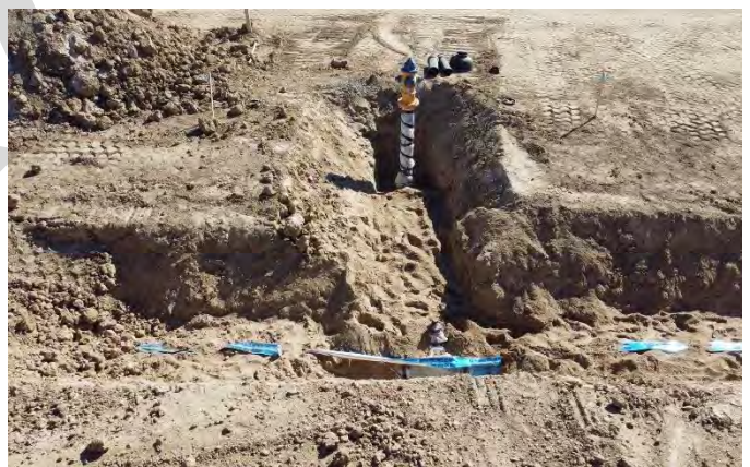
Filing 5 Wet Utility Improvements
