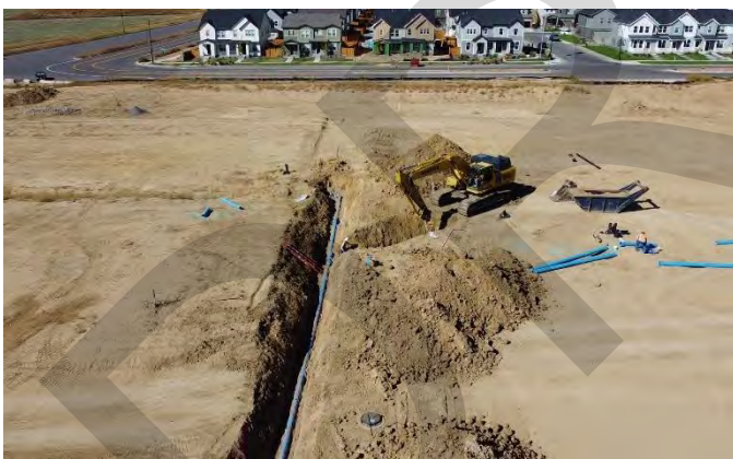
Filing 5 Wet Utility Improvements
