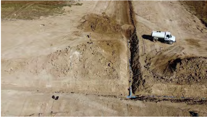
Filing 5 Wet Utility Improvements
