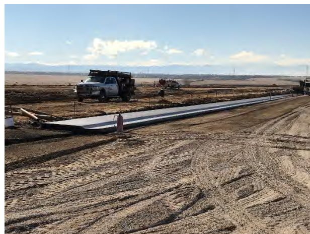
8 th Ave west of White Crow Street – curb and gutter and subgrade prep
