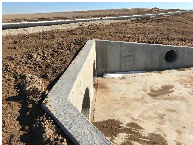
Storm Crossing Structure Monaghan Road north of 10 th Drive west side
